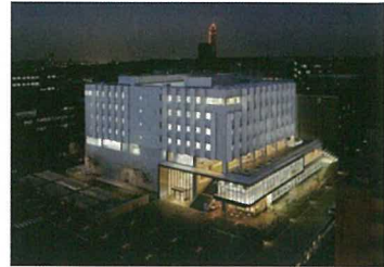
図6 施設の外観 Fig.6 An external view of the facility.
