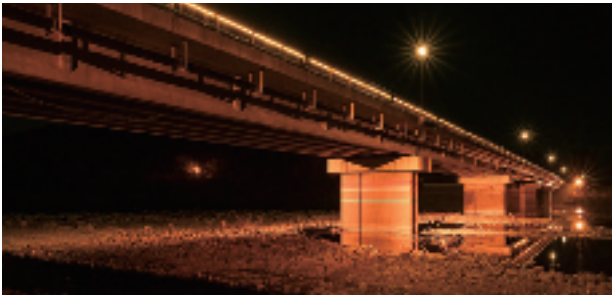
図8 河川内遊歩道から見た橋脚(平常時) Fig.8 Bridge piers seen from the river promenade (normal times).
