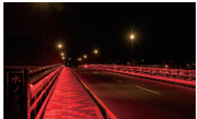
図7 橋上の様子(アラート時) Fig.7 Situation on the bridge (at the time of alert).
