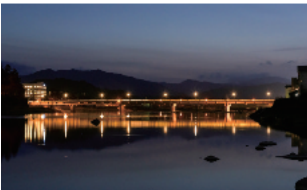
図5 上流からみた水の手橋(平常時) Fig.5 Mizunote Bridge seen from upstream (in normal times).
